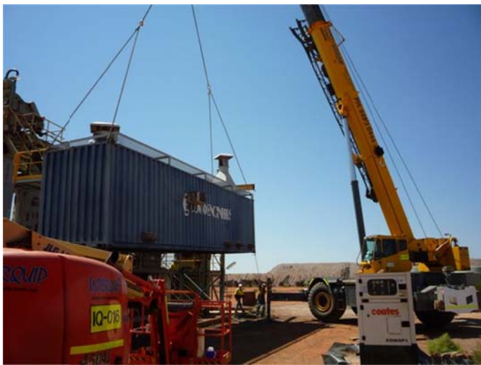
Fig. 1 Gold Room being removed from the Indee Plant
