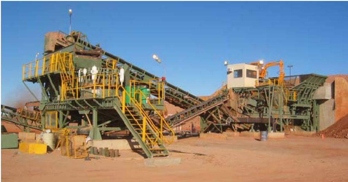
2 Stage Crushing Plant
