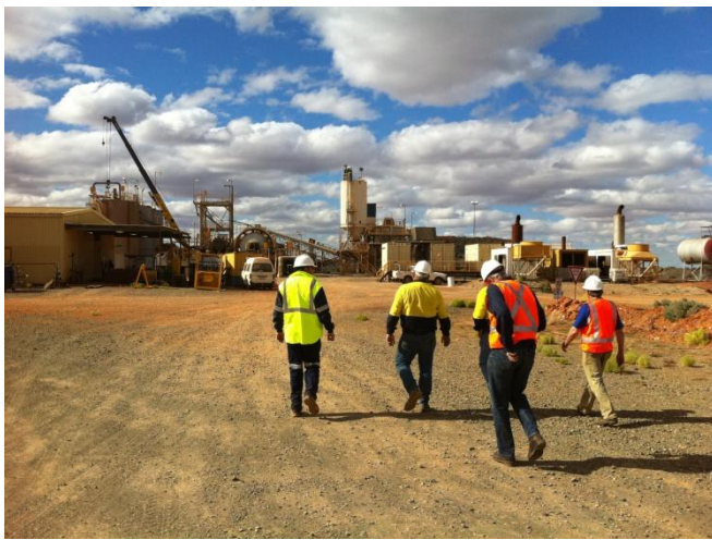
Burnakura CIL treatment plant, October 2011
